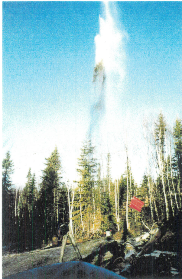
Figure 5: Example of dynamite blast from shot point 3
