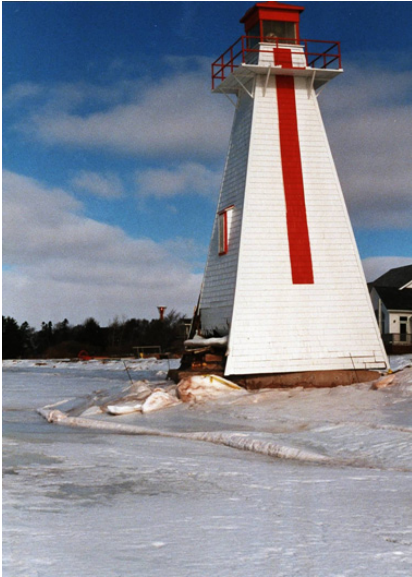
Figure 6. Damage to a Lighthouse in Charlottetown Harbour. The storm surge raised the water level above the foundation of the lighthouse and wind drove sea ice through the lower wooden wall and shifted the entire structure off its foundation. A sheet of ice can be seen protruding from the wall.
