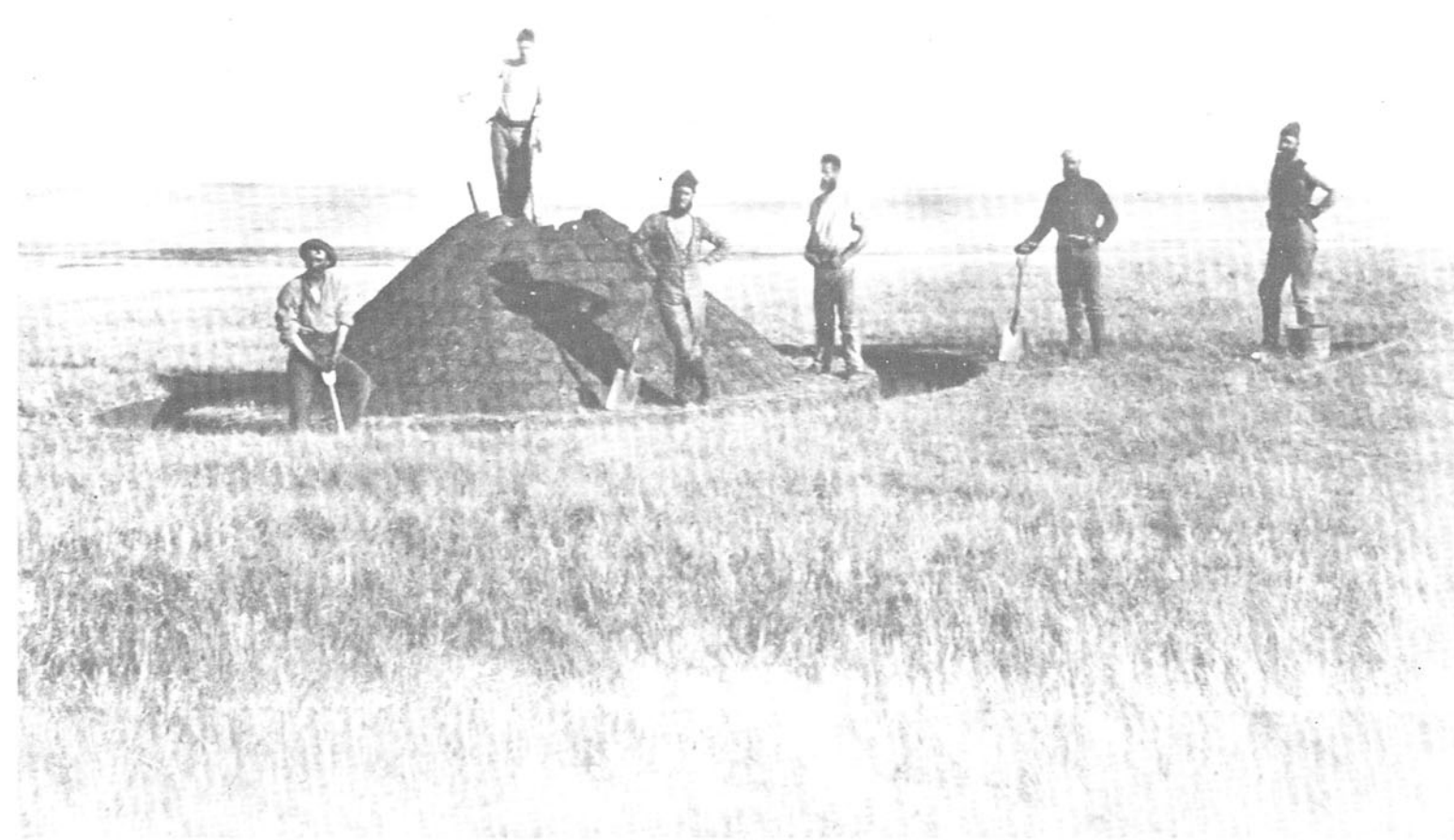
BOUNDARY COMMISSION 1873 — Supporters of the North American Boundary Commission building a "boundary mound" in 1873. These mounds marked the 49th Parallel and thus indicated the limit of jurisdiction of the U.S. Cavalry to the south and the North West Mounted Police to the north.
