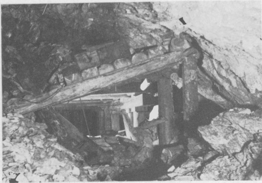
Fig. 56 Rockburst of January 29, 1943; 3908W Drift, looking west from Sec. 7W.
