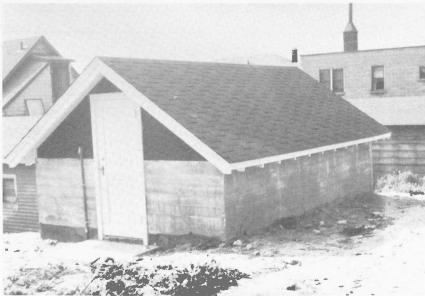
Fig. 81 Permanent Seismograph Vault at Kirkland Lake.
