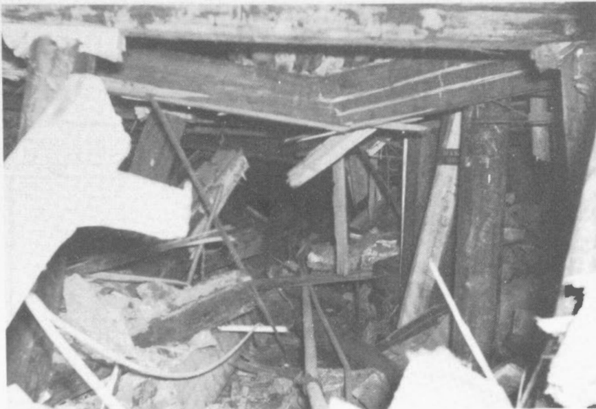
Fig. 57 Rockburst of January 29, 1943; 4001W Drift, looking west from Sec. 6.7W.
