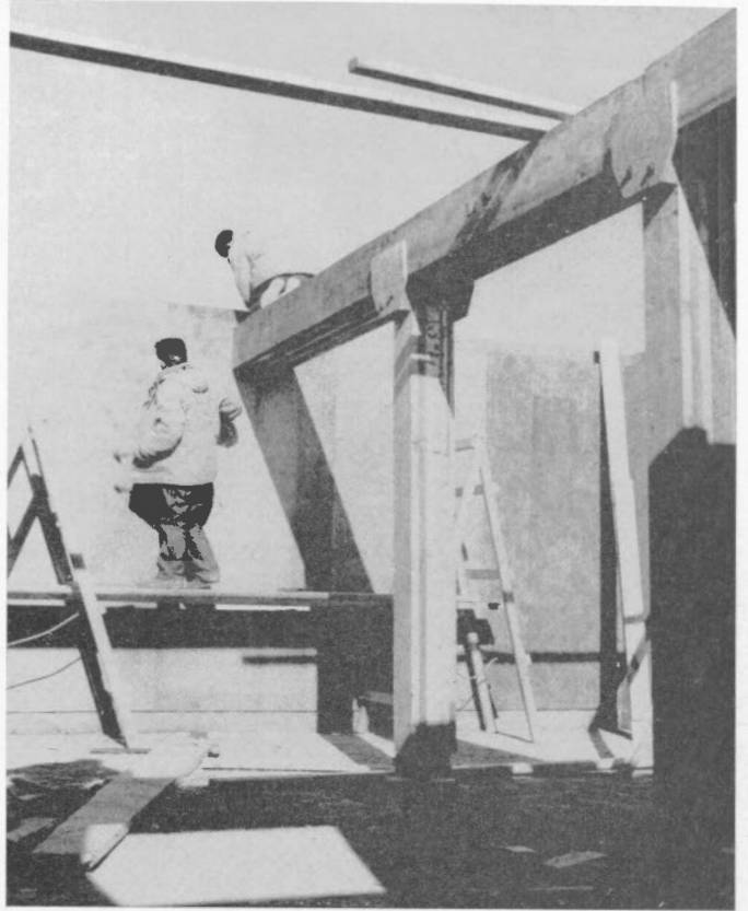
Figure 2. Interior view of construction.
