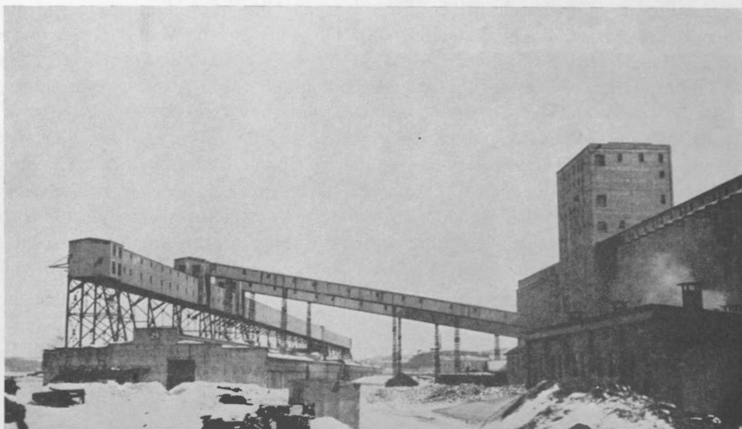
FIG. 7.—Grain elevator and freight sheds at Quebec
