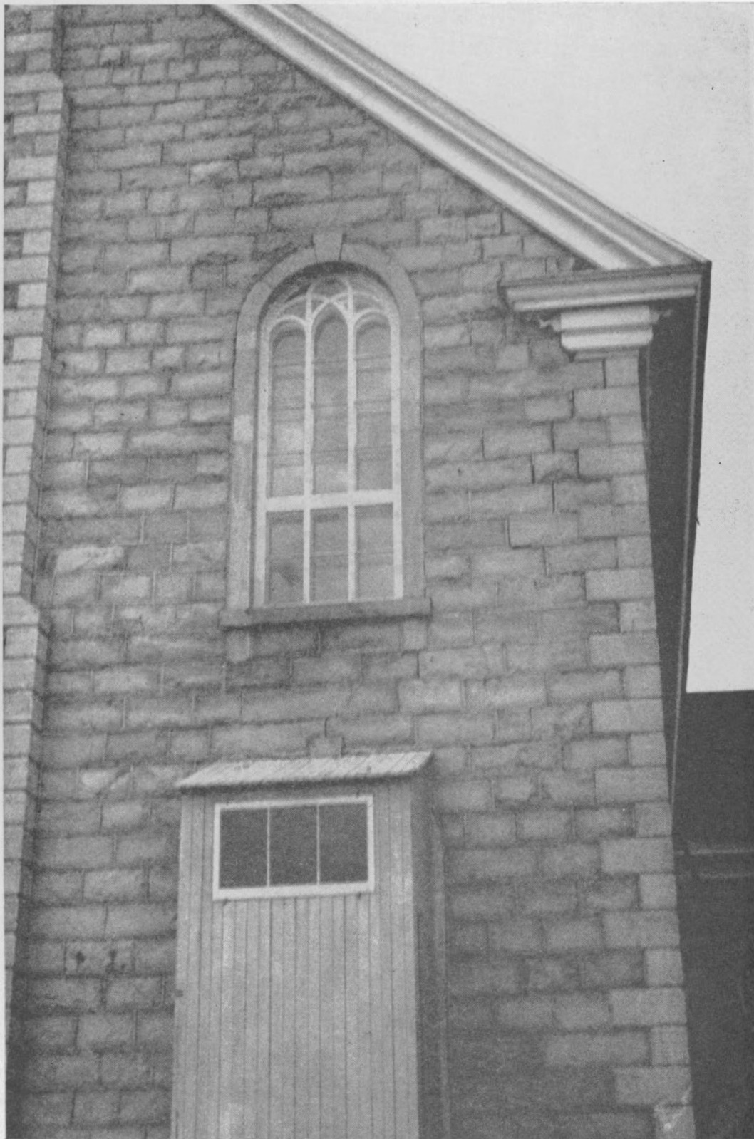
FIG. 3.—East side of front of Rivière Ouelle church
