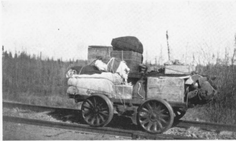
FIG. 2. TRANSPORTATION ON HUDSON BAY RAILWAY Railway motor lorry on which the magnetic survey party made the trip from The Pas, Man., to the end of steel, a distance of approximately 330 miles.
