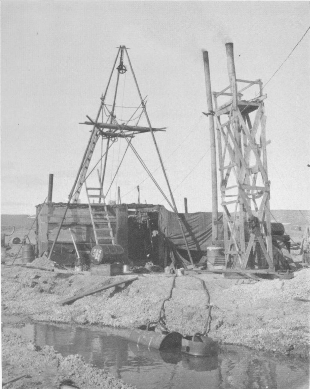
FIGURE 2.—Drill set-up showing tripod and two coil water heaters.
