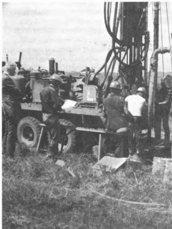
Drilling for lignite in Saskatchewan. Dr. D. S. Montgomery Energy Research Program Director observing operations
