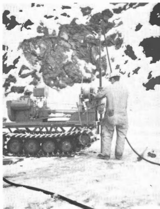
Prototype diamond drill developed under contract.
