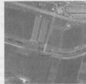
Figure 11. A bridge not on a gravel area in a river stream
