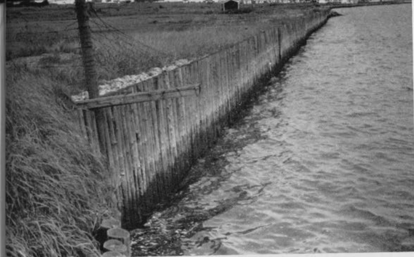
Figure 13. An example of a pile retaining wall in good condition.
