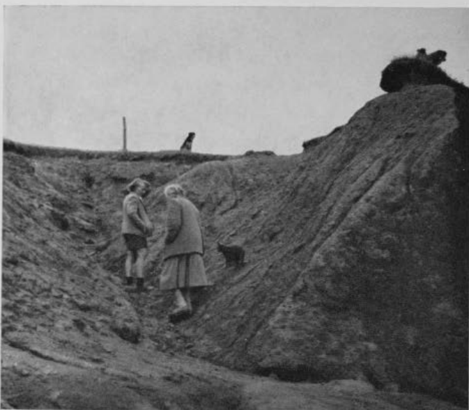
Figure 5. A large gully has been cut by running water in the unconsolidated material of a sea erosion face.
