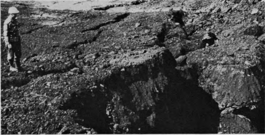
Figure 7. Much of the energy of the blast in permafrost is absorbed by the ice segregations. Here a poor blast has resulted in incomplete rupture of the pit back wall. June, 1960.
