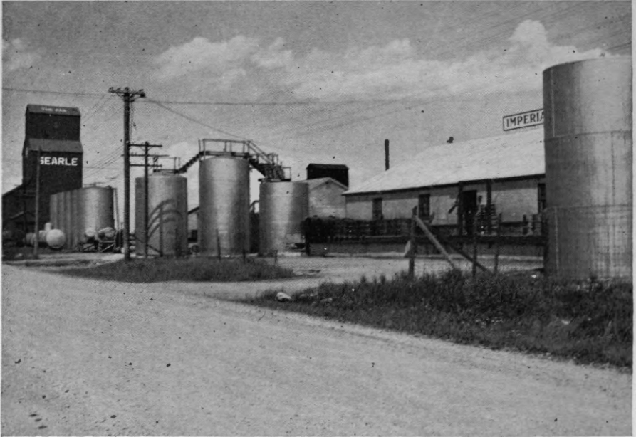
Figure 8. British American and Imperial Oil storage tanks at The Pas, Manitoba. Note the Searle Company grain elevator in the background.
