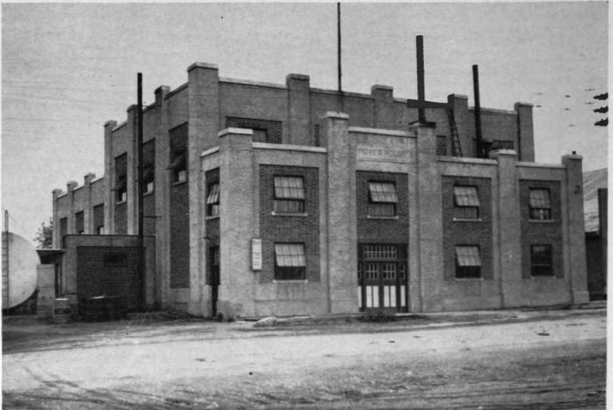
Figure 14. Power house and pumping station at The Pas, Manitoba.
