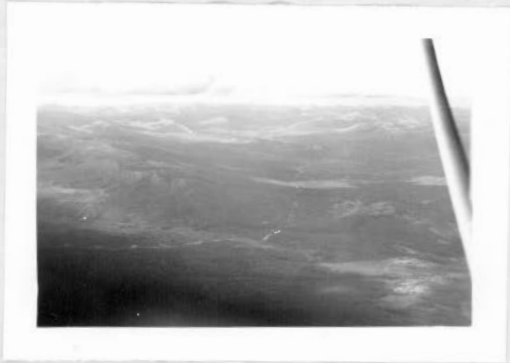
Oil pipe and highway near Teslin.
