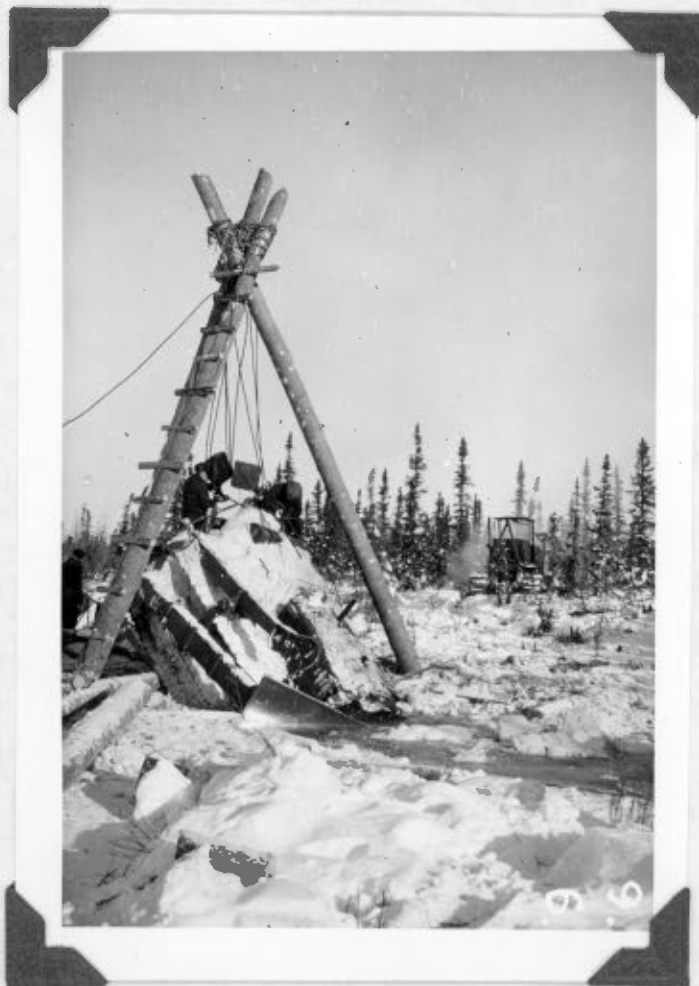
Transferring cable onto drawbar to lift bulldozer higher.
