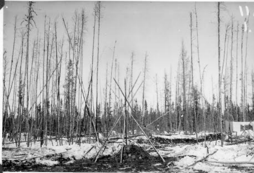
Complete station mark, looking north along loop in trail.
