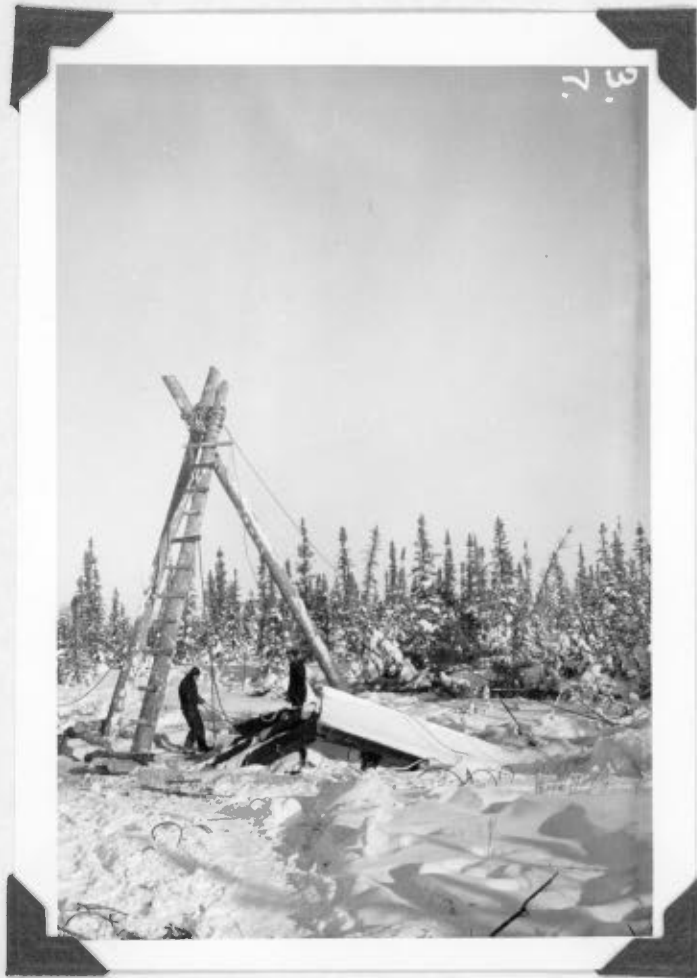
Tripod of 20 ft. timbers erected over TD 18
