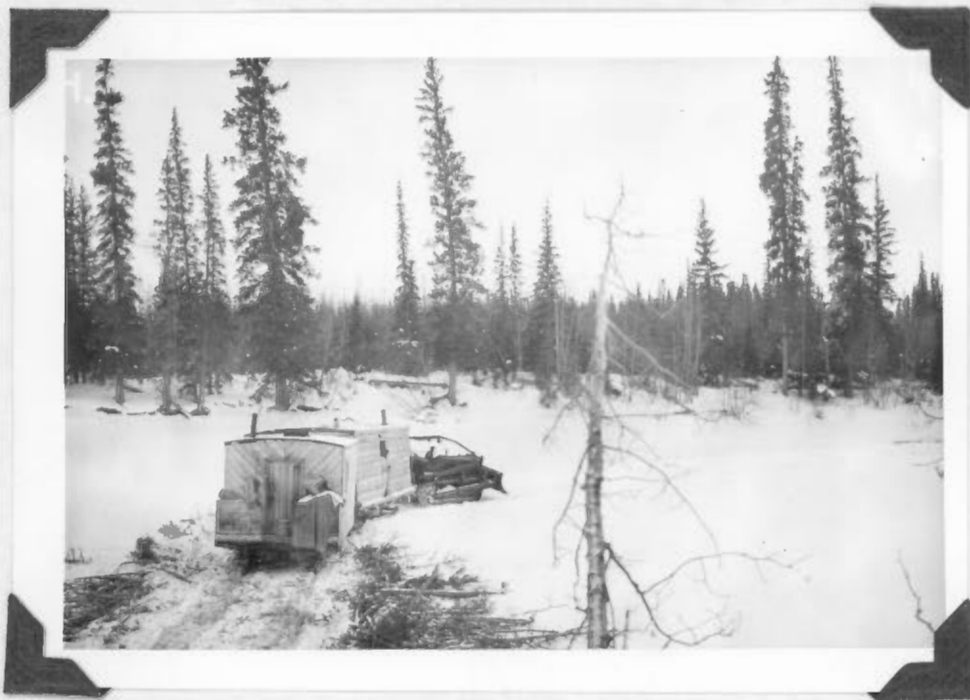
Tractor train crossing Whitesand River. Note ramp of brush and snow down river bank.
