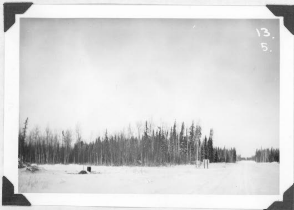
Looking north along Mackenzie Highway, showing station marker at left.
