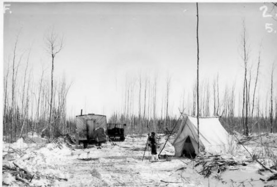
Observing tent and theodolite, looking east along trail before station mark erected.
