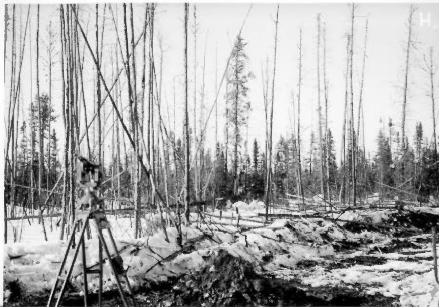
Theodolite and incomplete station mark, looking northwest.
