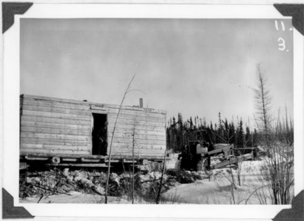
Tractor train crossing unfrozen sulphur stream. Note the bridge of brush and snow across stream.
