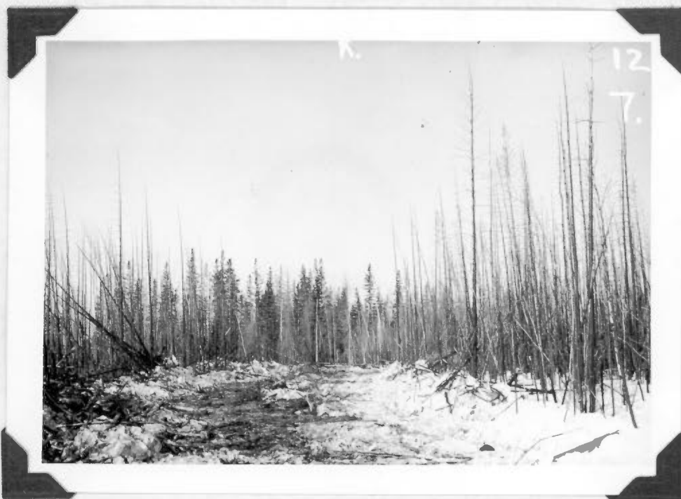
Station marker, looking west along loop-back in trail.
