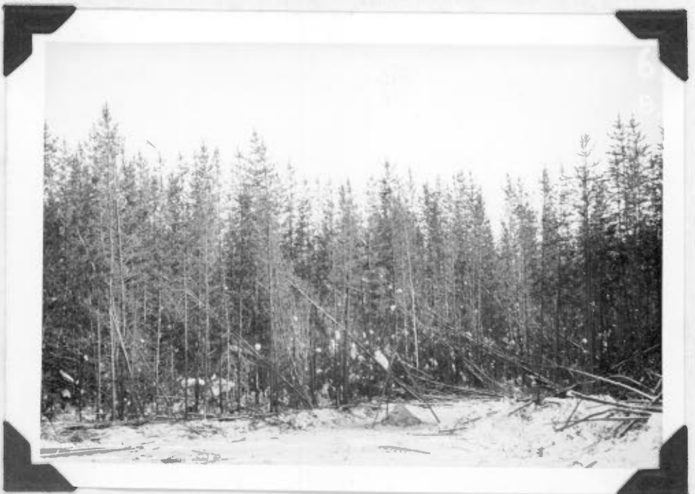
Looking south of east at completed station mark.
