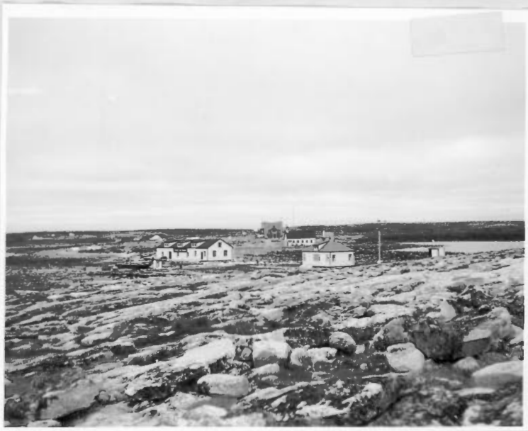
H.B.C. Post at Chesterfield R.C. Mission in background.
