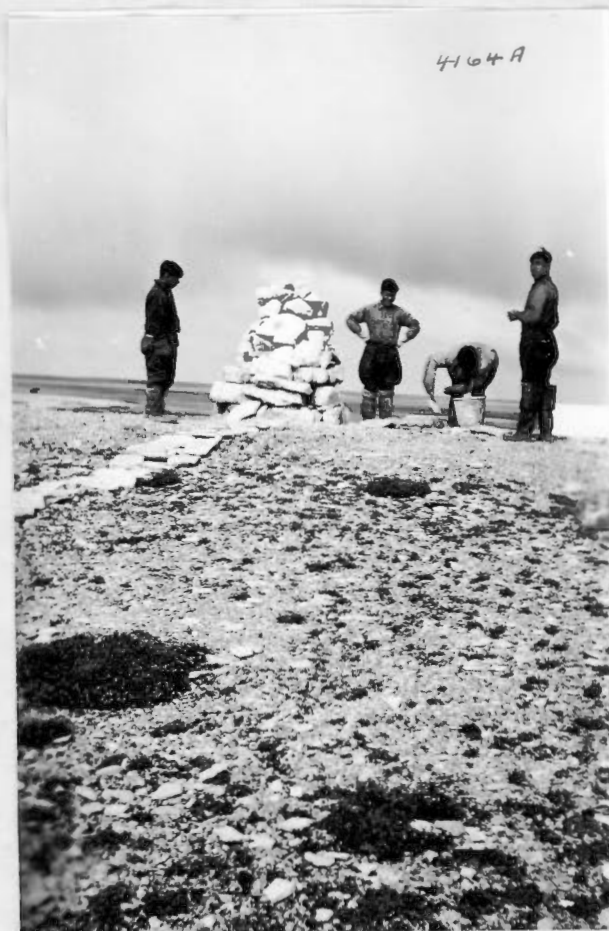
At Cape Low, Southampton Island our Eskimos are whitewashing strips of flat stones. These make the point easily seen from the air and when photographed serves to identify the survey mark with the surrounding topography. Below we see the markings as photographed at 2,000 feet.
