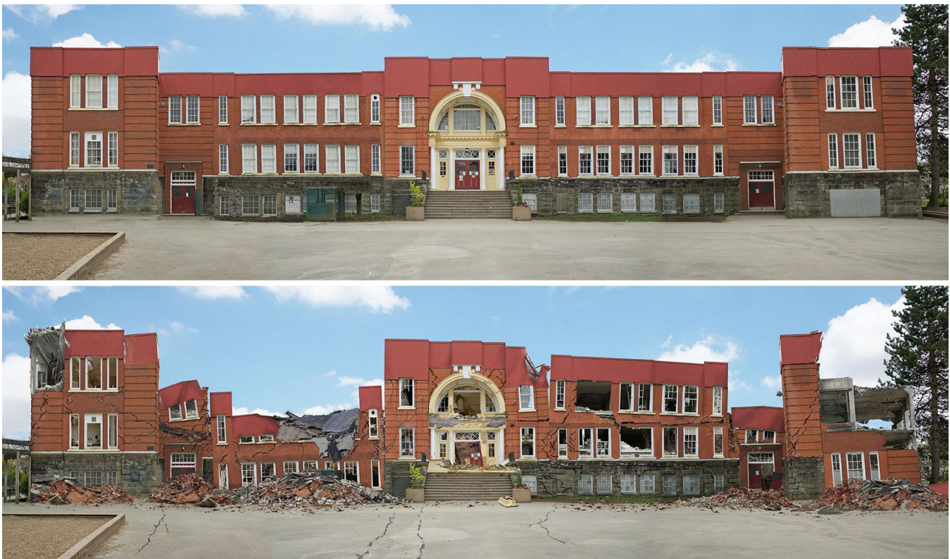
Figure 4: Artist illustration of potential earthquake damage at an elementary school in Vancouver (Photo/illustration: UBC News).
