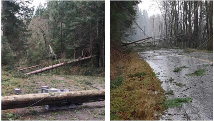
Figure 2: Fallen trees and poles during 2018 windstorm (Photos: BC Hydro).
