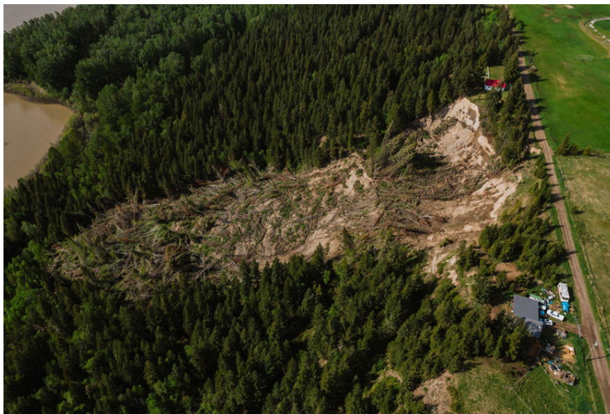
Figure 3: Church Road slide at Highway 97, May 17, 2021. The spring freshet resulted in flooding and damage at over 90 road sites in the Cariboo (Photo: flickr/Ministry of Transportation and Infrastructure).
