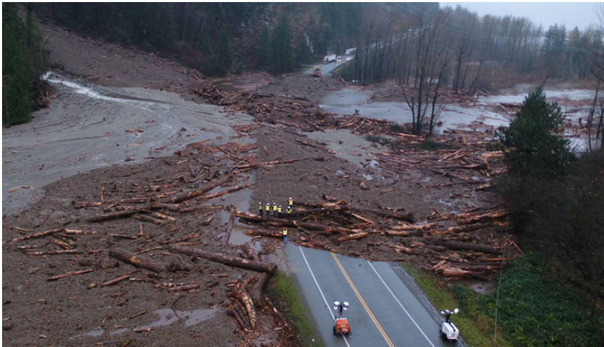
Figure 2: Assessing damage at Ruby Creek and Highway 7 after mudslide closes the road, November 15, 2021 (Photo: flickr/Ministry of Transportation and Infrastructure).
