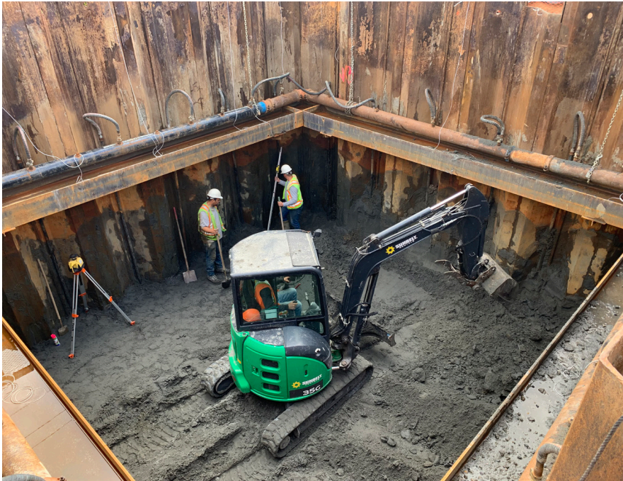
Figure 1: Construction of a new pump station (Photo: NDMP).
