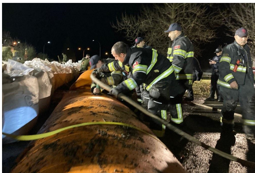
Figure 6: Inflatable flexible tubes set up during the November 2021 flood (Photo: BC Ministry of Transportation/flickr).
