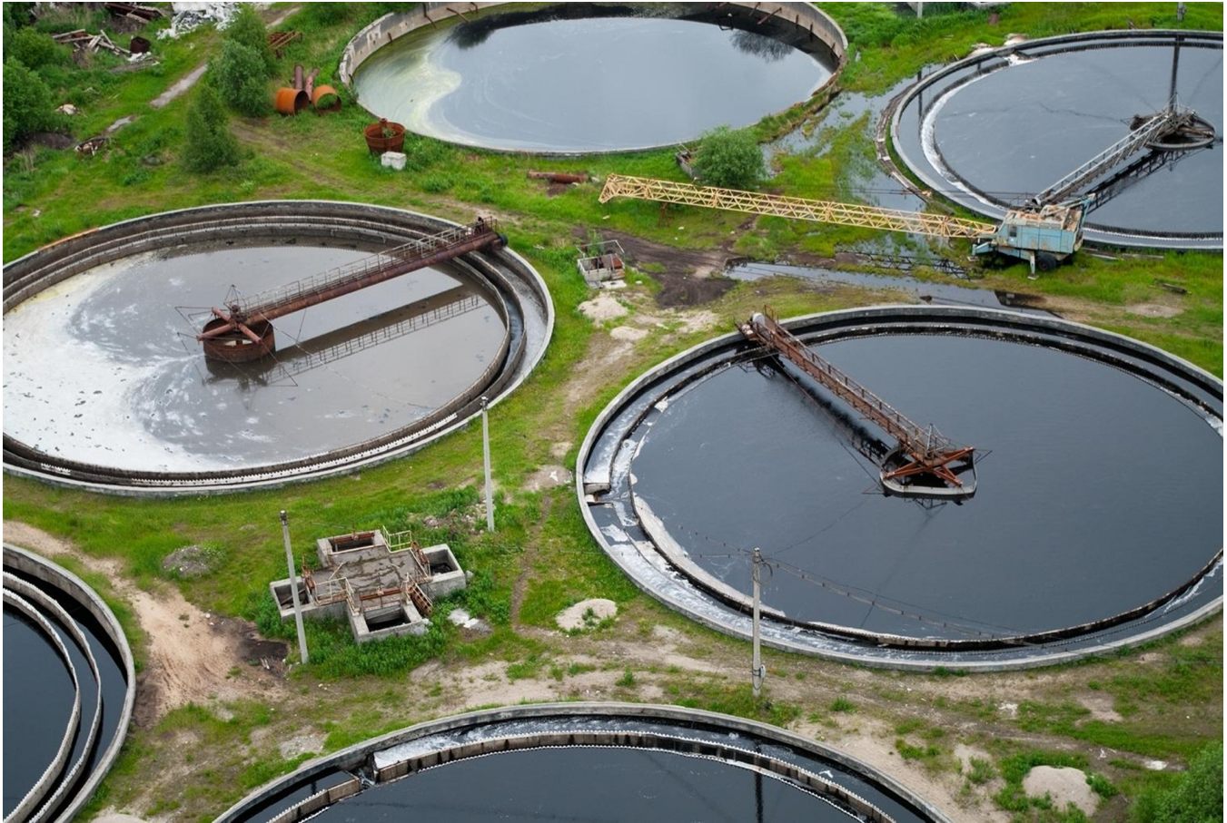
Figure 2: Wastewater treatment plants provide critical water infrastructure (Photo: Public Safety Canada).
