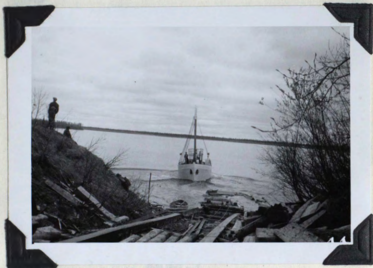
Looking N. W. of the schooner as it is on the way down the launch to the water.
