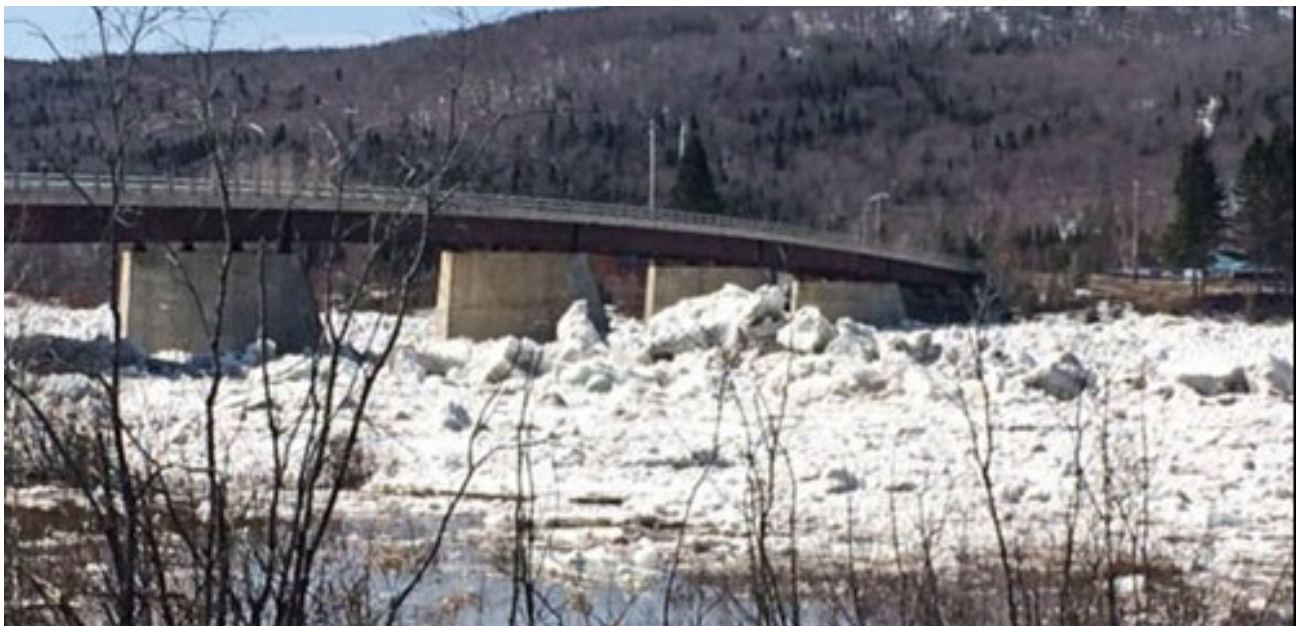
Figure 10: Spring ice jam at a rail bridge on the Saint John River. (Source: New Brunswick Power, 2015)
