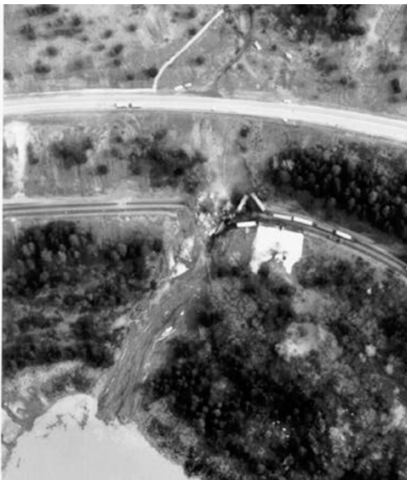
Figure 13: Conrad, British Columbia train derailment. Collapse of the railroad subgrade was caused by extreme precipitation. (Source: Transportation Safety Board of Canada)
