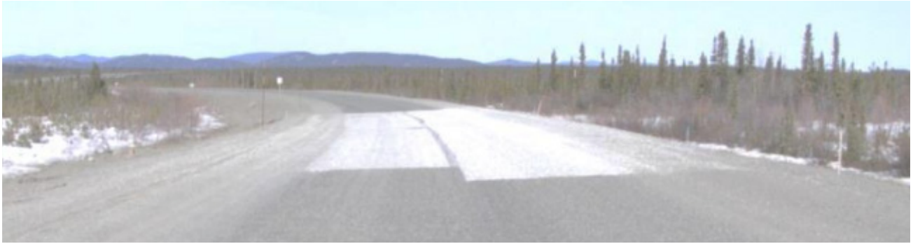
Figure 11: Test section of high-albedo (light-toned) surface treatment. (Source: Paul Murchison)
