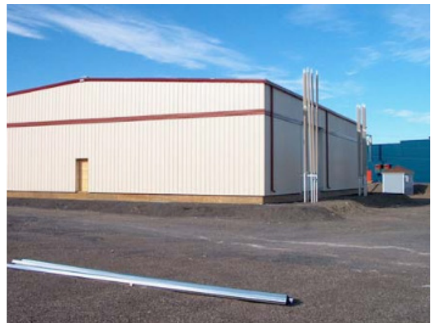
Figure 13: Flat-loop thermosyphon foundation at an airport maintenance garage in Inuvik, NT. (Source: Igor Holubec)
