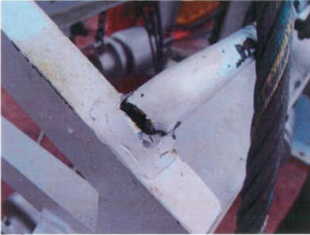
Broken steel bar at the top of the air gun sled.
