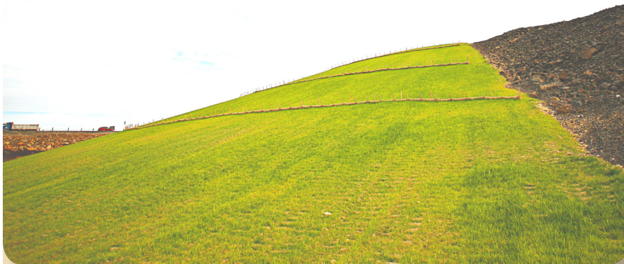
Partly revegetated slope of slag pile shows before (right) and after (left) effects of regreening. Photo courtesy of Vale.
