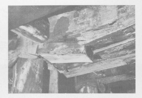
Fig. 10 Beam Broken by End Thrust.
