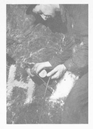
Fig. 64 Loading Geophone into Borehole.
