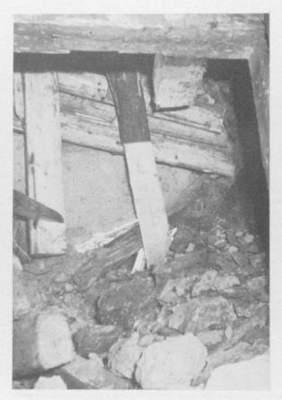
Fig. 54 Rockburst of January 29, 1943; 3801W Drift looking west from Sec. 6.5W.
