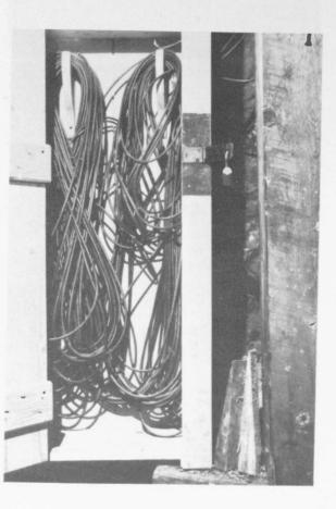
Fig. 72 Cable Reservoir; 4700-ft Level.
