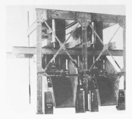
Fig. 14 Loading Pocket at Discharge Bins.
