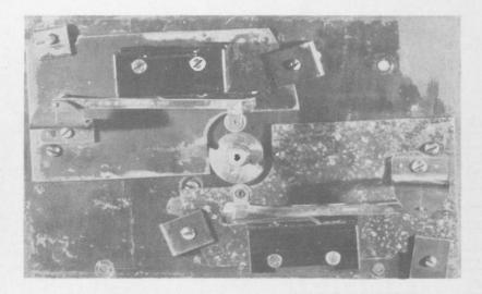
Fig. 67 Alternating Switch; Quadruple-line Recording.
