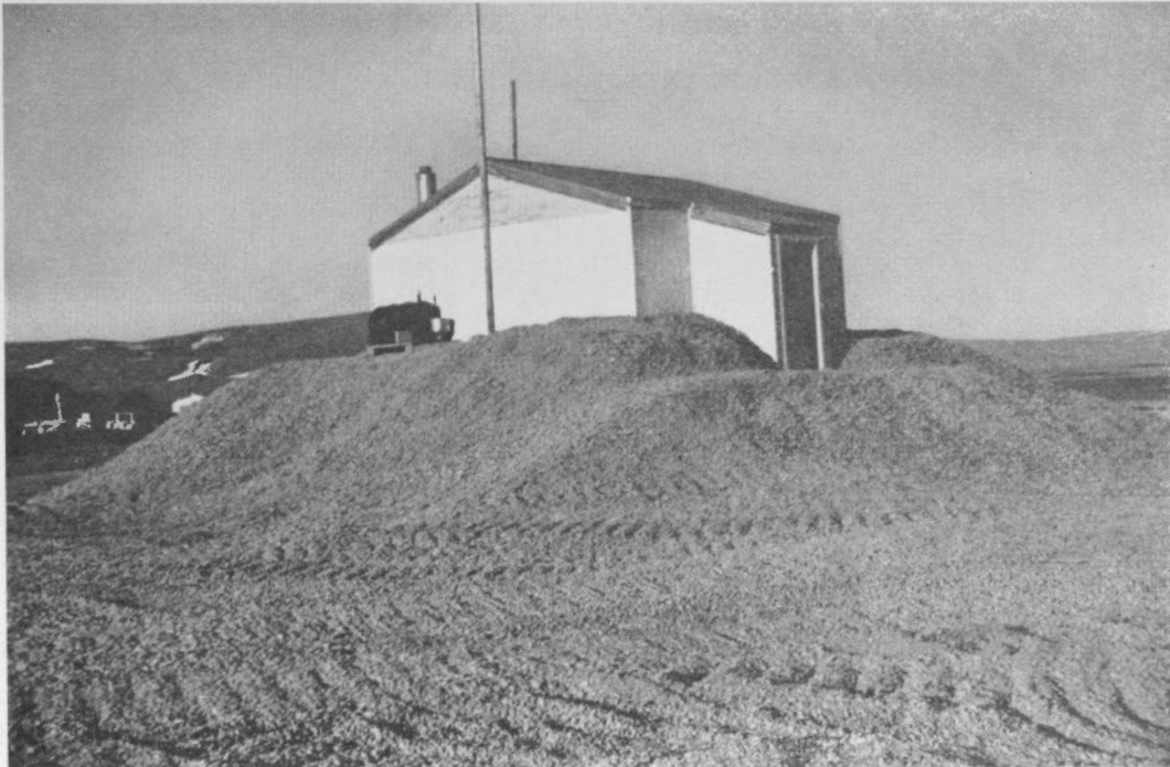
FIGURE 8—Recorder building completed. Note the oil reservoir and chimney of the oil-fired space heater.
