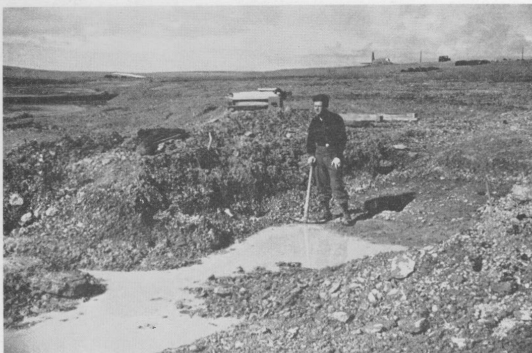
FIGURE 1—Excavation through permafrost to expose bedrock for seismometer shelter.
