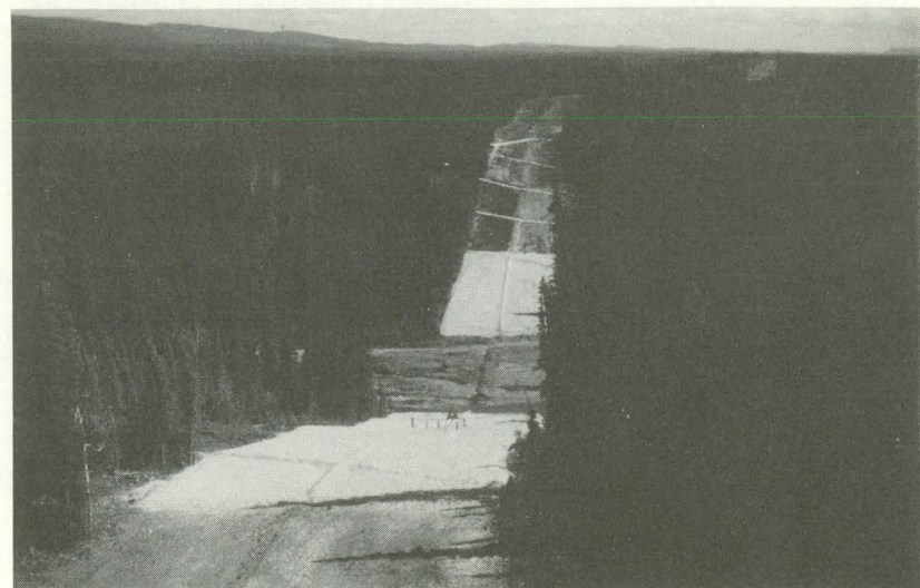
Erosion control berms on the north side of Bear Rock, near Fort Norman (June 1984).
