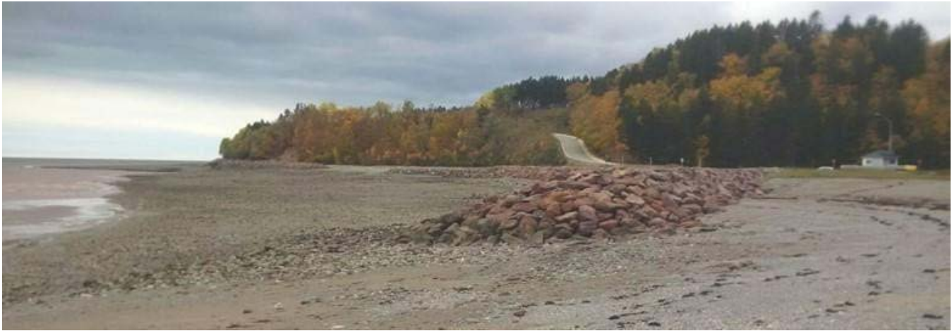
Figure 1.4: Rock revetment, combined with beach openings, used to protect the highway embankment at the entrance to Fundy National Park in Alma, New Brunswick, at low tide. Photo courtesy of Doug Watson, Parks Canada.
