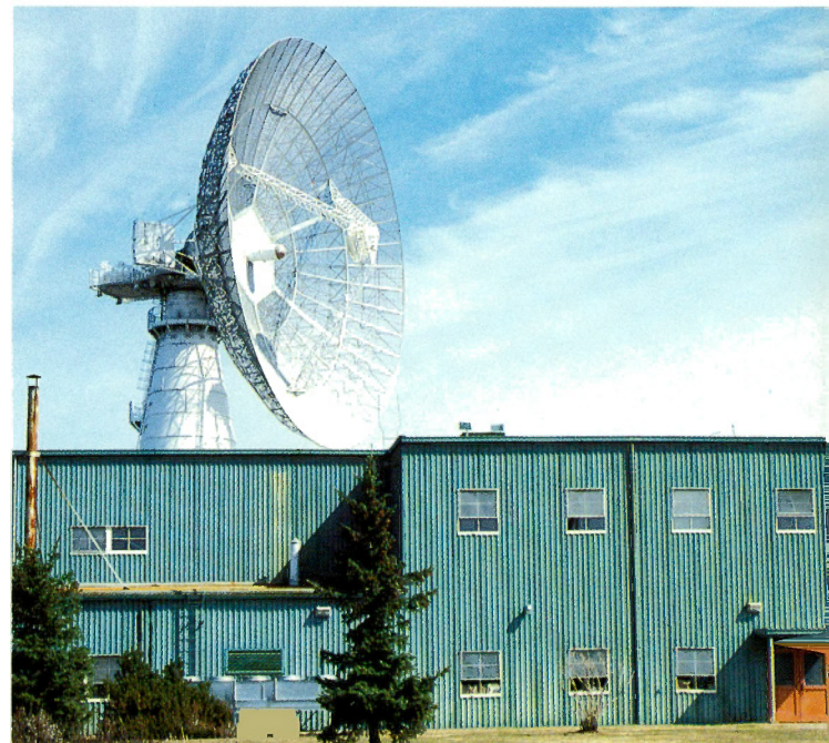
Receiving Station, Prince Albert, Saskatchewan
