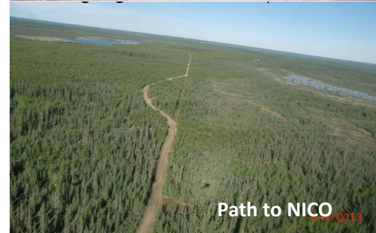
All weather Tłıchǰ Highway and winter road
