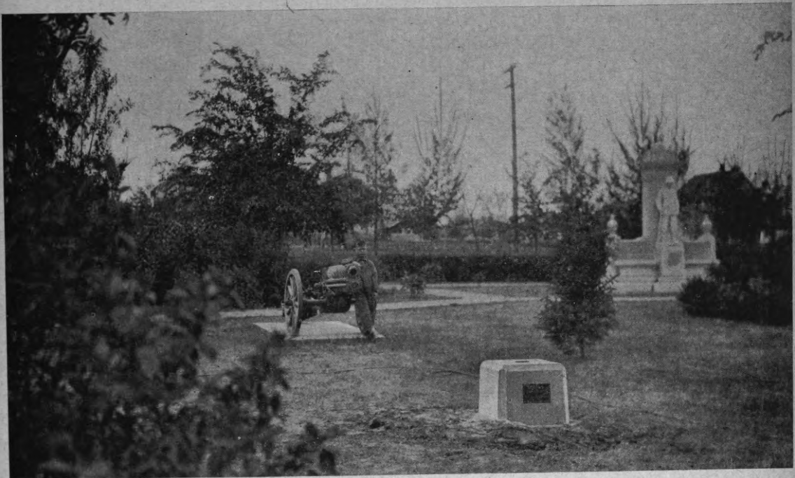
Fundamental Bench Mark Pier in Memorial Park, Assinibota, Sask. The bench mark is a bronze tablet, three inches in diameter set in the top of the monument. On a bronze plate on one face of the monument is inscribed the elevation of the bench mark above mean sea level.
