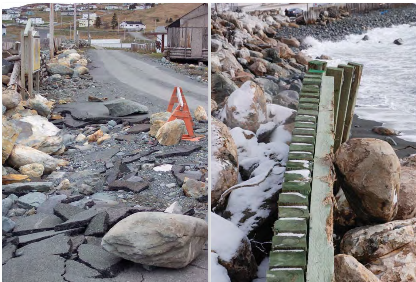
Figure 3: Storm damage, 2004 (Left), temporary wooden barrier, in place after storm in Dec. 2009 (right).
