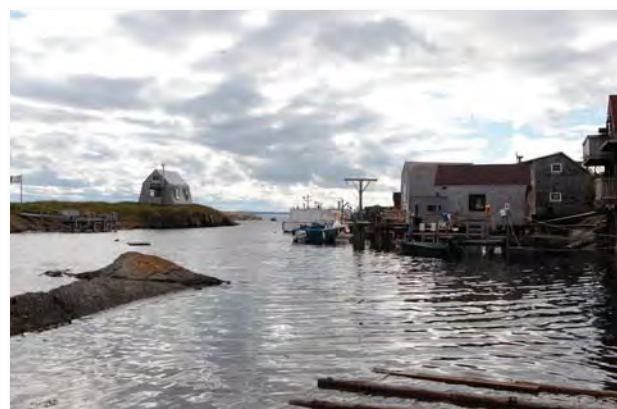
Blue Rocks, like many MODL communities, has much of its infrastructure directly along the coast.
