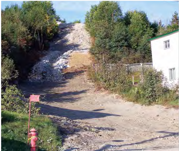
Figure 2: Remedial measures – Humber Road, Riverside Drive area, Corner Brook. The city installed a storm drain (lighter disturbed ground to left) following a slope failure triggered by a single rain-on-snow event in March 2003.
