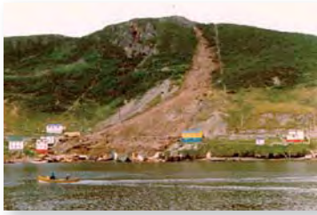
Martin Batterson, Debris flows - In 1973, a debris flow destroyed four houses in Harbour Breton, NL.
