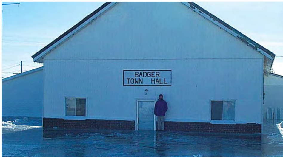
Photo credit: Water Resources Management Division, Department of Environment and Conservation, NL
