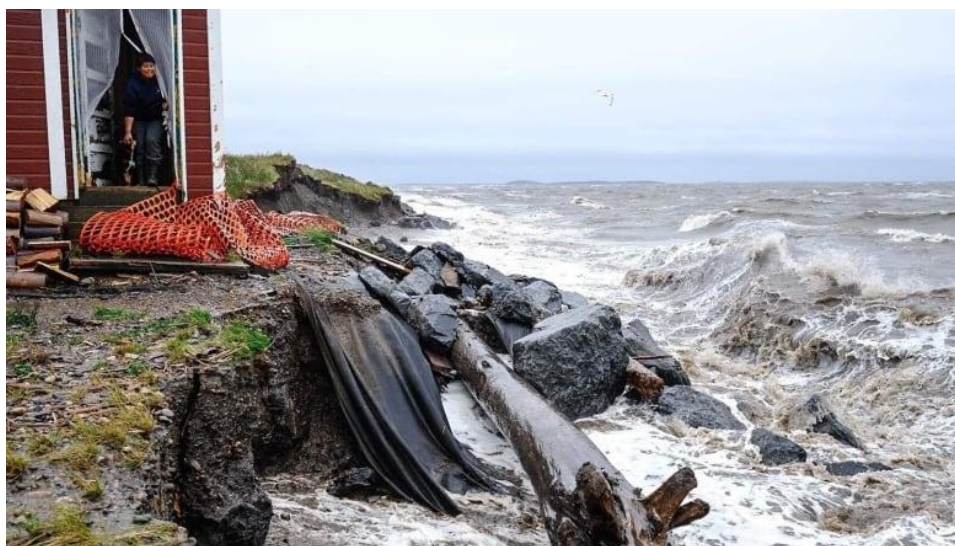
Figure 11. Makeshift coastal barriers to protect from erosion in Tuktoyaktuk 9
