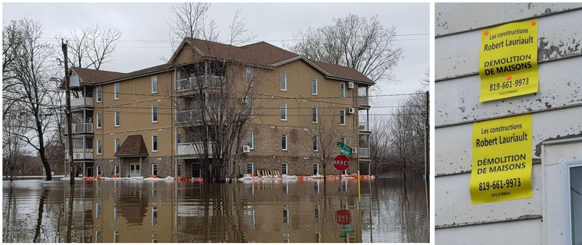
Figure 9. Flooded condominium and post-buyout home demolition signs 7
