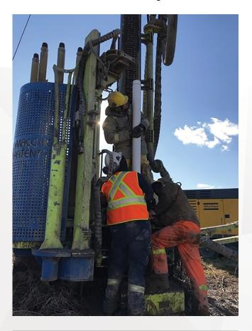
**Figure 13.** Observation well installation in the Vars-Winchester esker near the city of Embrun in Ontario.
