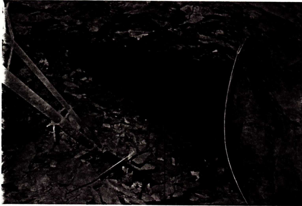
Damage to a sill drift at the Quirke Mine.
