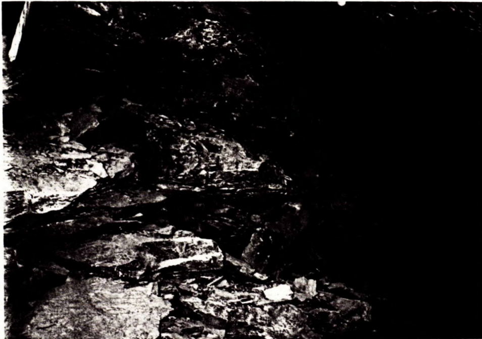
Over 800 tonnes of displaced rock due to two small (2.0 Mn) rockbursts in an isolated haulage drift at Strathcona Mine.
