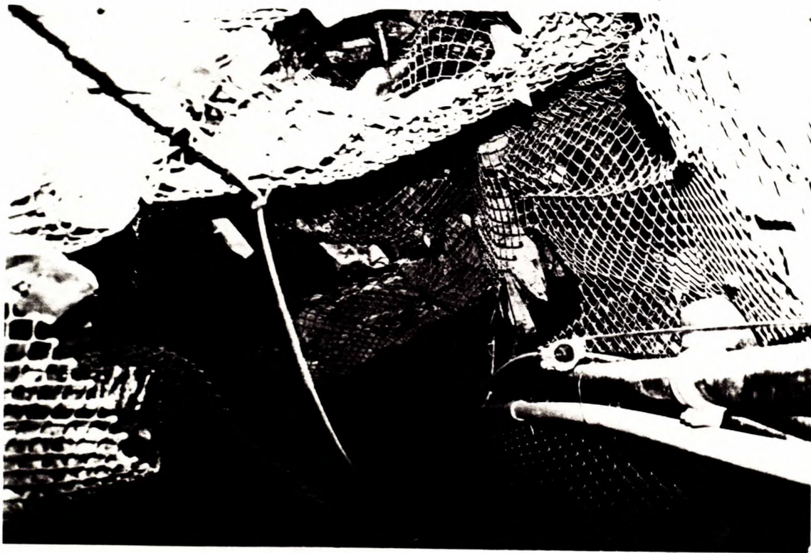
Damage from a 3.1 Mn rockburst at the Macassa Mine. Bolts and chain-link mesh prevented complete closure of the drift.
