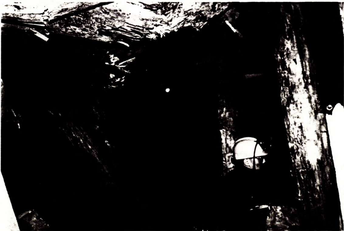
Rockburst damage to a drift supported by timber posts and beams at the Macassa Mine.
