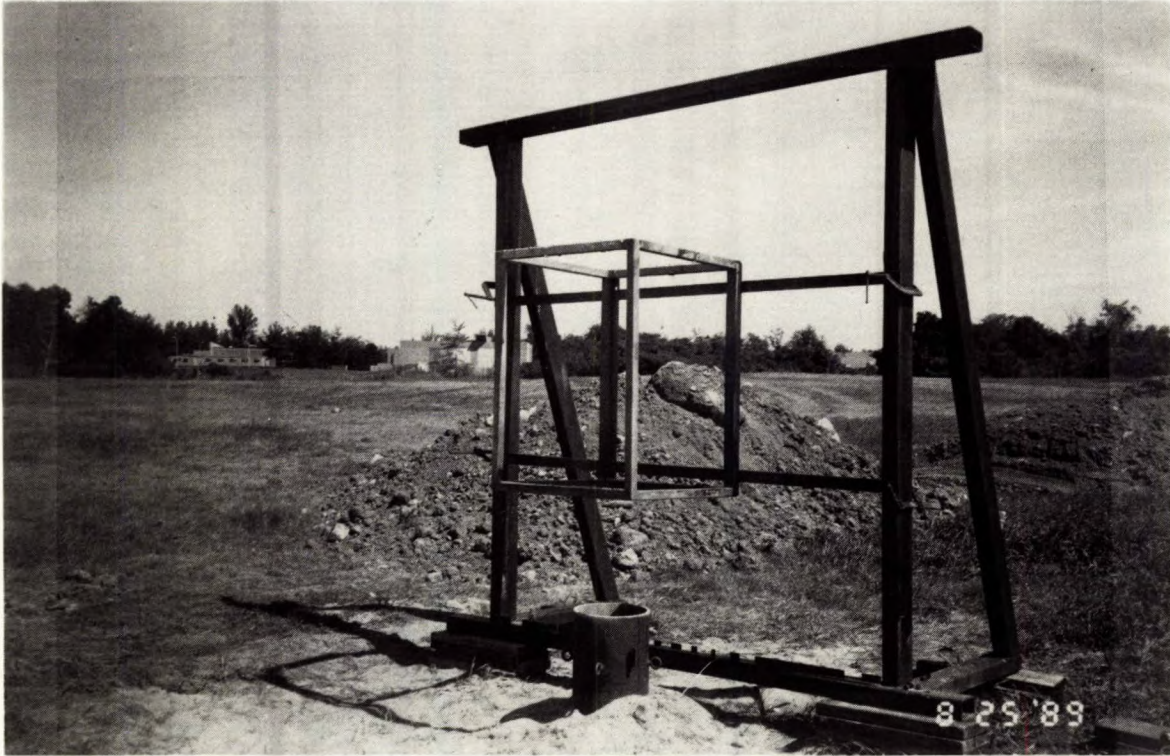
Fig. 3 - Short mortar set-up
