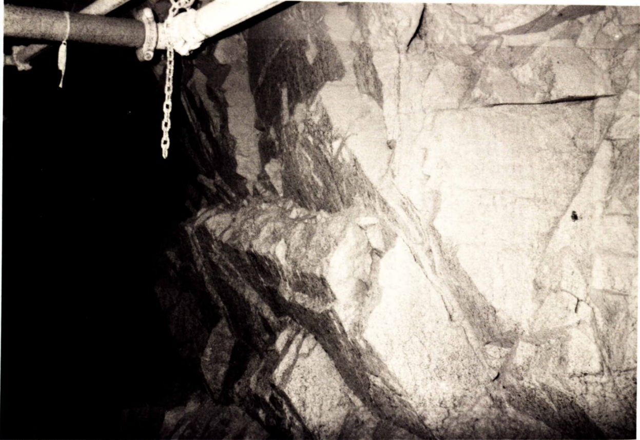
Figure 11 Potential side wall toppling failures. The opposite wall would be subjected to sliding failures.
