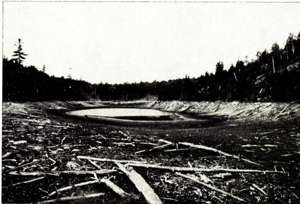
Hanging wall above a rockburst area fractured through to surface causing disappearance of a small lake.
