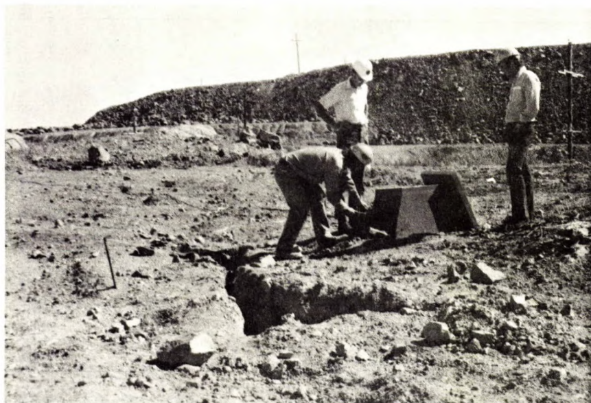
Figure 1. Automatic Crack Monitor, Endako, August 1975
