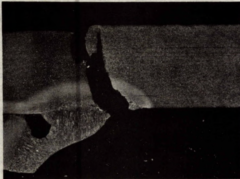
Figure 8 - Section B4 (See Figures 3 and 5) showing path of fracture close to the toe of the fillet weld joining the connecting plate (lower left) to the inner surface of channel B.
