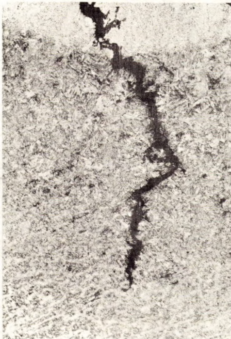
Figure 8 - Extremities of brittle crack in relatively sound section of fillet weld around patch.
