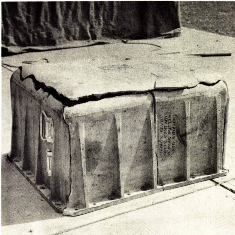
Fig. 2. - Another view of the broken cover shown in Figure 1. One face has broken in half. It is probable that failure started at the corner nearest the camera.
