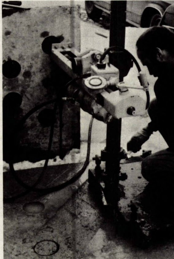
Fig. 3 - A view of the cores being drilled from columns.
