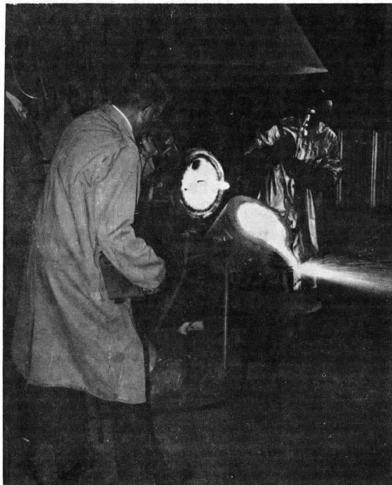
Figure 3 - Blowing mineral wool
