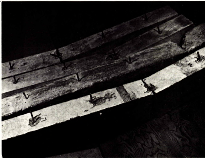
Fig. 6 - A view of the 6 x 6 x 66-in. test beams after probing.
