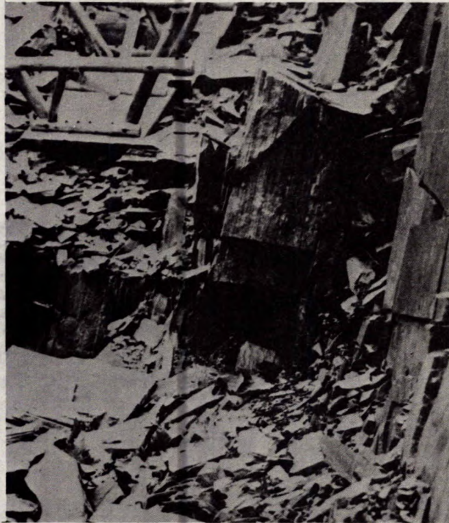
Figure 4. View of cleavage characteristic of rock in the area. Large quarry (compare size of slabs with overturned picnic table).
