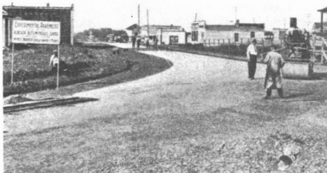
Bituminous sand pavement laid by S.C. Ells in Edmonton, 1915
