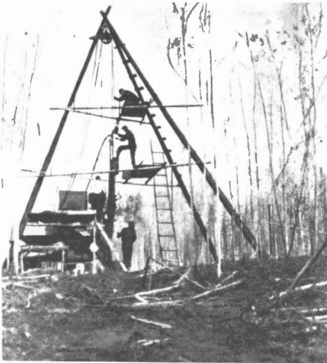
Drilling for bituminous sand in the Steepbank area, Alberta
