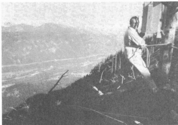
F. Kapeller installs control box for extensometer used in monitoring stability of large B.C. open pit mine coal
