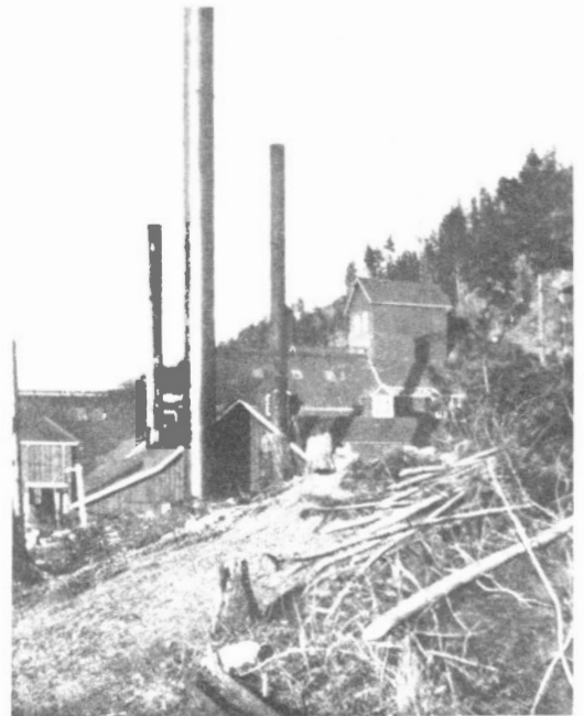
Boiler house, Sullivan mine, B.C., circa 1905
