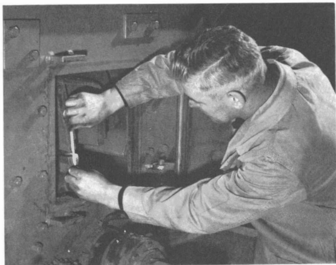
A. Boissonault adjusts impact crusher before treating northern Ontario iron ore
