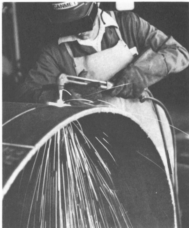
M. Letts cuts test sample from large diameter commercial gas pipe
