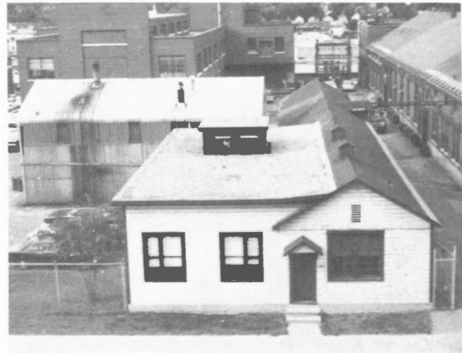
Electrical Certification Laboratory (554 Booth St.) 1954, on site of old machine shop; new machine shop (556 Booth St.) is at left rear; Butler building for carbonization studies is in middle rear
