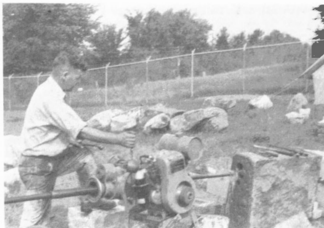
L. Richards drills rock samples in connection with jet-piercing research project at Uplands
