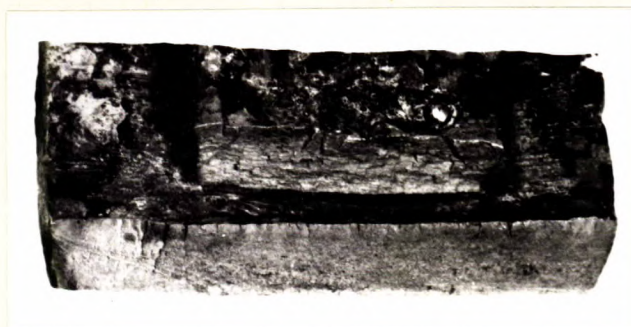
PHOTOGRAPH SHOWING SMOOTH, BRITTLE FATIGUE FRACTURE OF RING (BOTTOM) AND FIBROUS FRACTURE OF REINFORCING PLATE (TOP).
