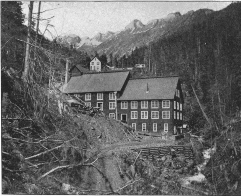
WHITEWATER MILL.—Whitewater, Ainsworth, B.C.
