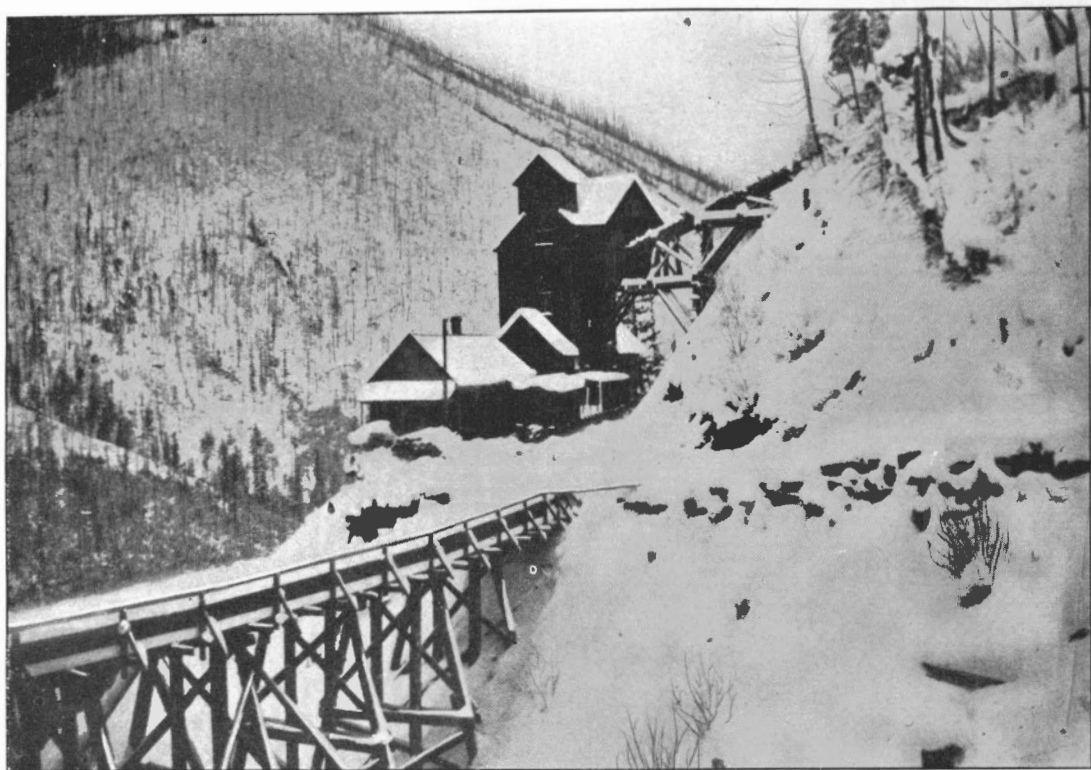
VIEW OF THE PAYNE LOWER TRAMWAY TERMINAL.
