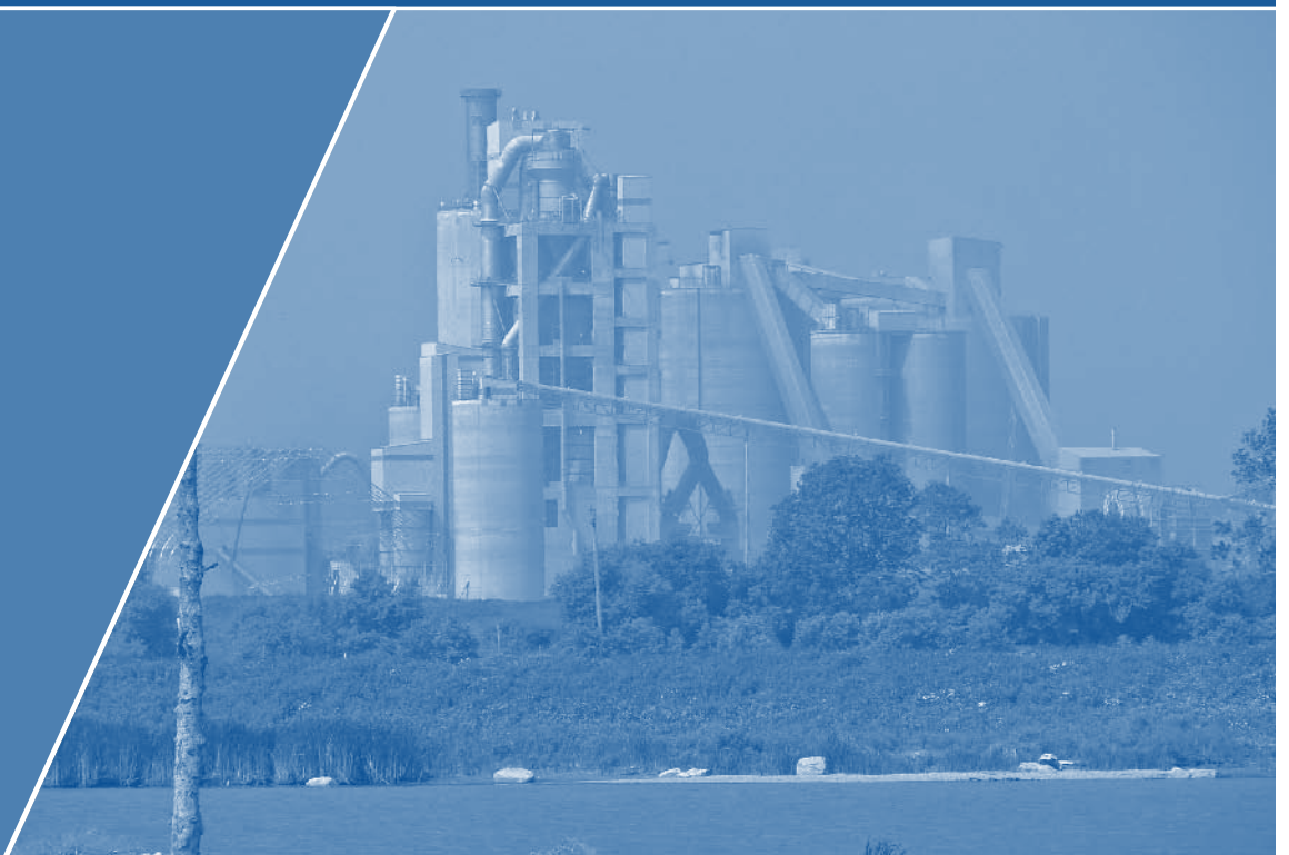
St Marys Cement Bowmanville plant from the West Side Creek Marsh Conservation Area, Ontario
