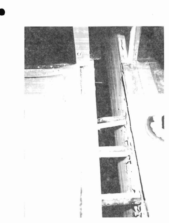
Figure 2. Compressional failure of rigid pipes containing wires, separation gap between 2 blocks of Whakatane Hospital building.
