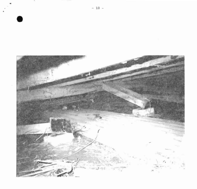
Figure 5. Failure of timber piles, house at Edgecumbe.
